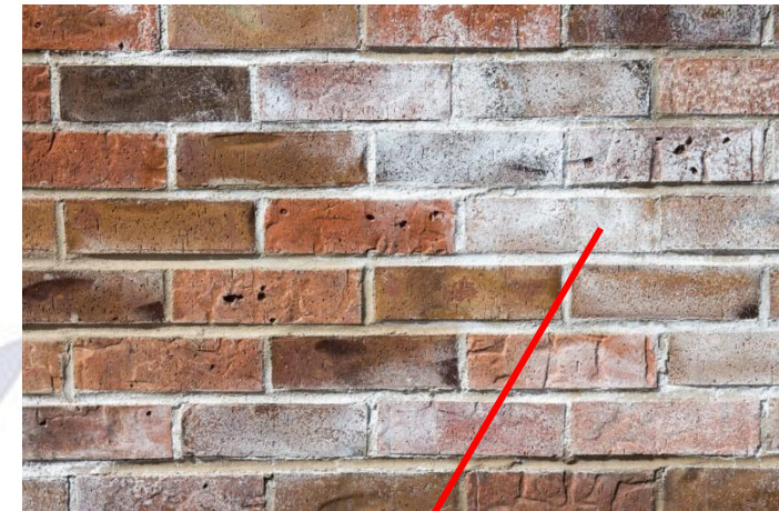
Efflorescence
